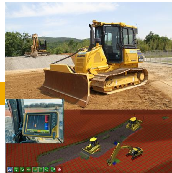
Directing the use of heavy equipment and performing remote troubleshooting
