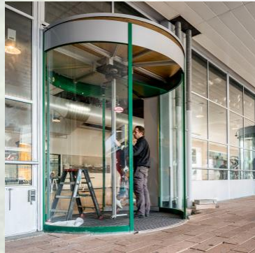
Refurbish old doors
